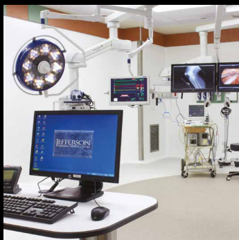
Signal Switching and Extension
