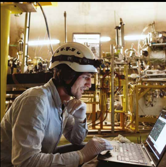
Redundant and Remote Networks
